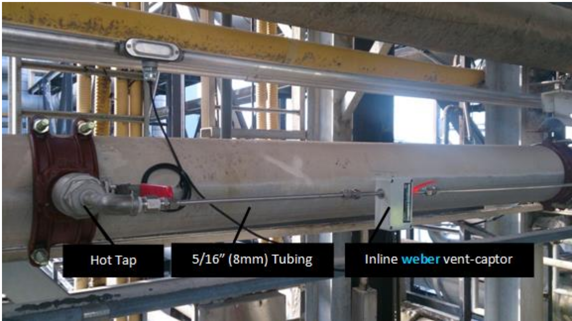
Installed vent-captor
